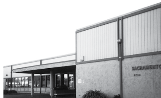
Sacramento County Office of Education Lincoln Village Drive building
